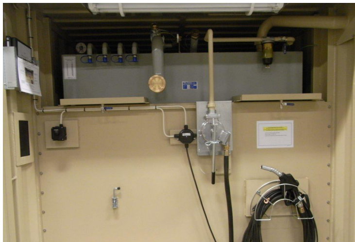
Collecting vessel with manual ATEX fillingpump
